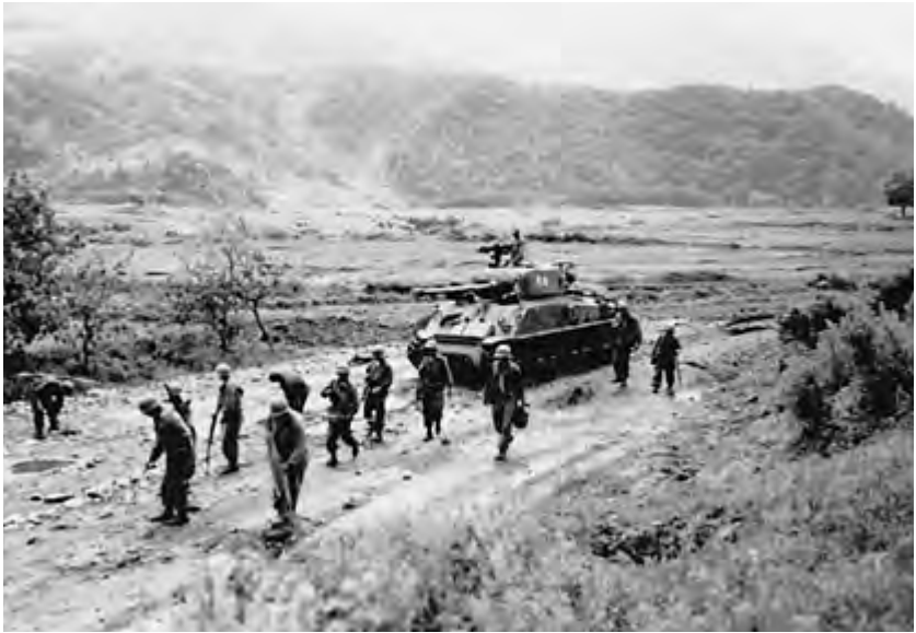
Engineers probe for enemy mines ahead of a creeping tank south of Ch'orwon, 10 June 1951. (National Archives)
